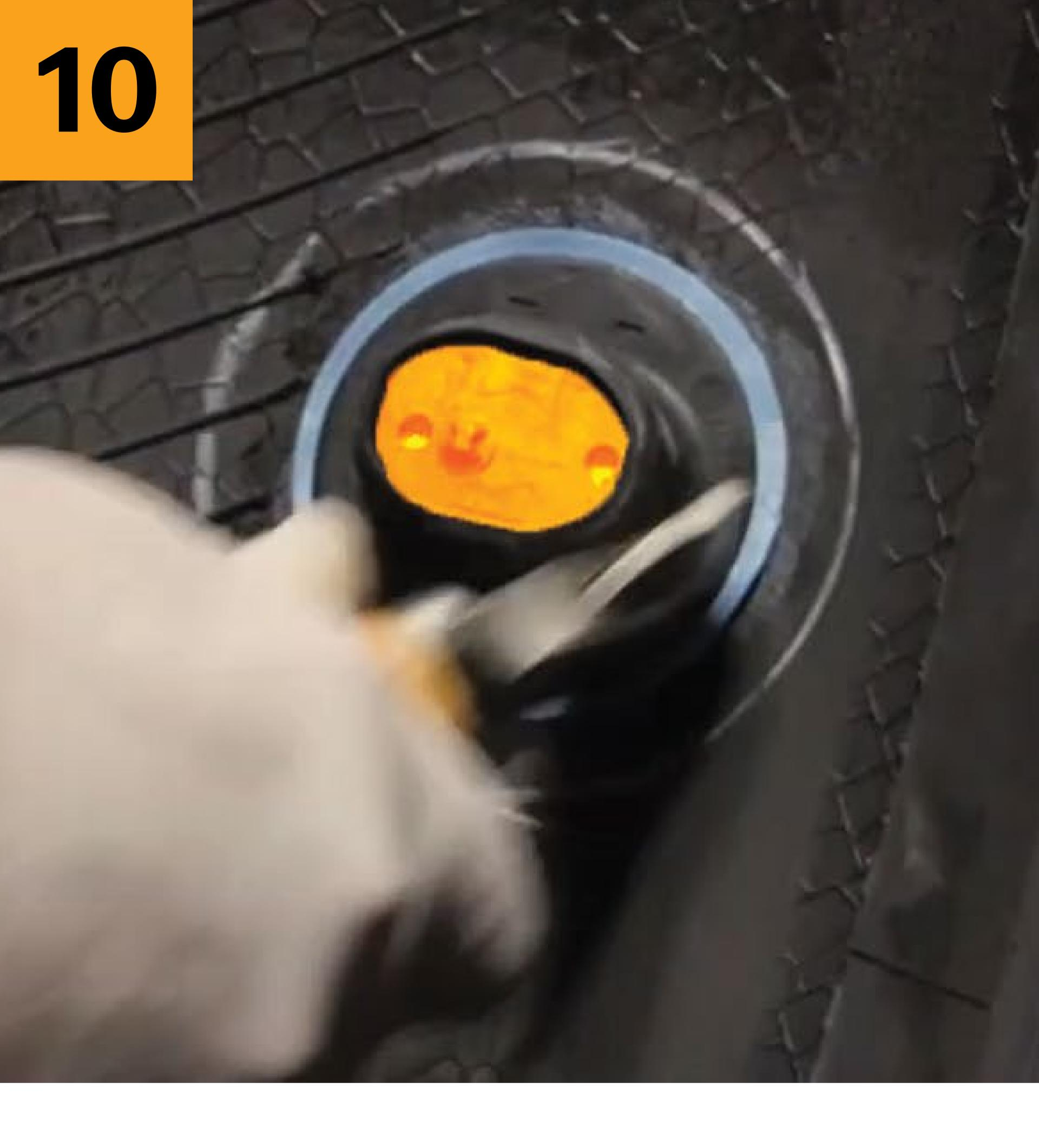
Remove any trapped air around the edges using the roller & stitcher.
